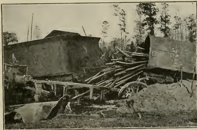
FIG. 1—RESULTS OF BOILER EXPLOSION DUE TO DEFECTIVE AND INSUFFICIENT CROWN BAR BRACES.
